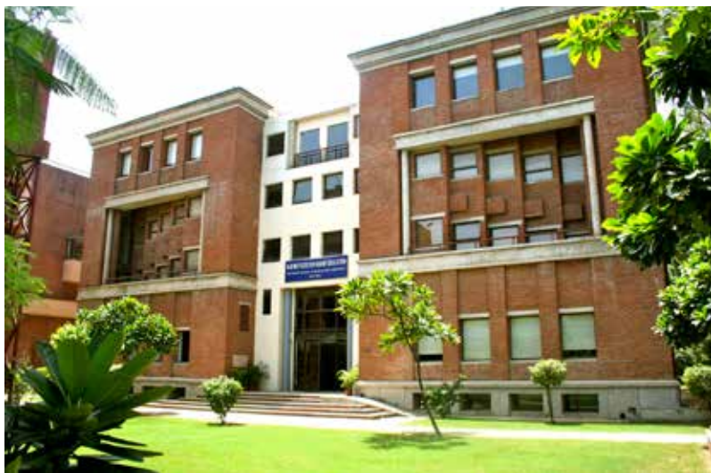
Lodhi Road Campus
